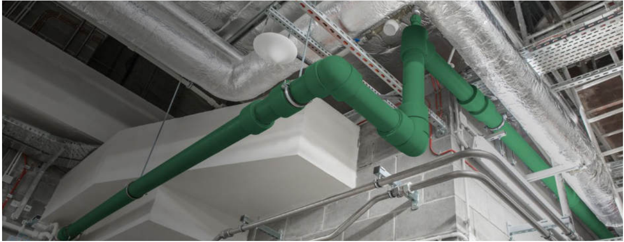
KAN-therm PP Green installation
