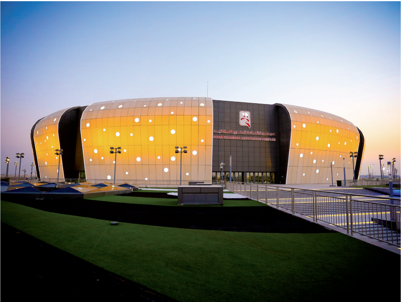
Qatar Handball Association Complex, Doha, Qatar
